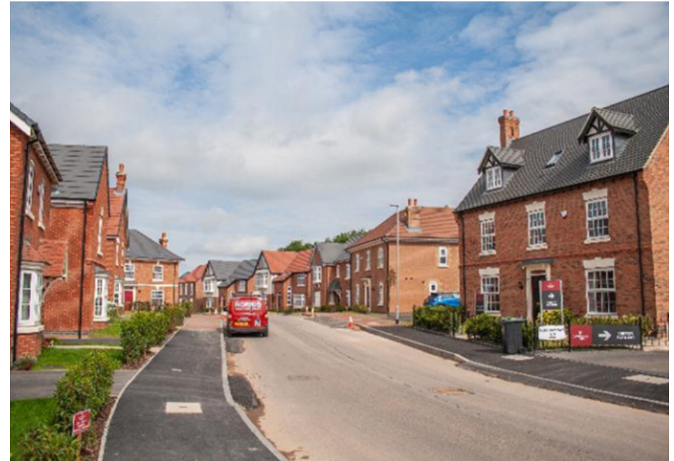
Figure 19: Whilst being built to a good specification, development employs a 'commercial' vernacular that expresses the housebuilder brand rather than reflecting local built forms. The images are from developments at Mapperley Plains.
